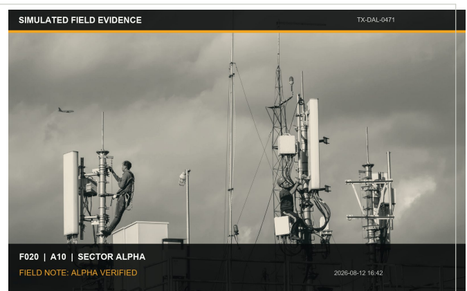
A10 | Alpha: Weatherproofing and final workmanship are visible
